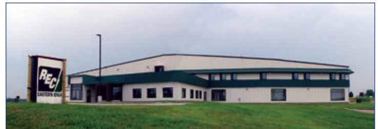
Eastern Iowa Light & Power Cooperative.
