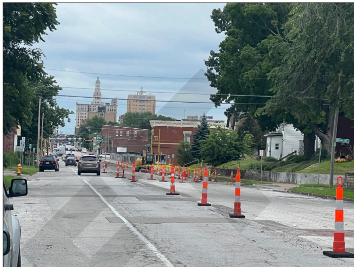
Figure 4.6 – Sample Road Construction, Davenport, Iowa
