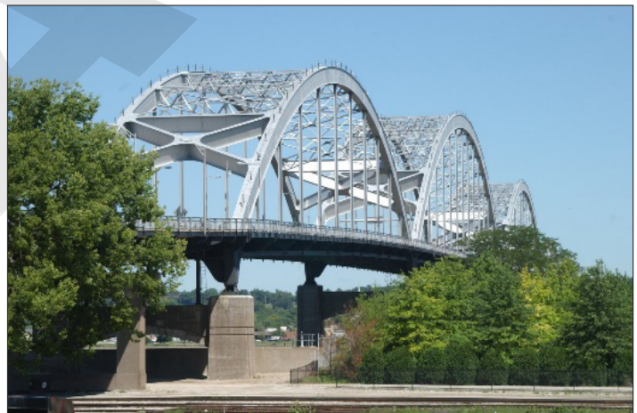
Figure 4.4 – U.S. 67 Centennial Bridge at Mississippi River, Rock Island, Illinois
