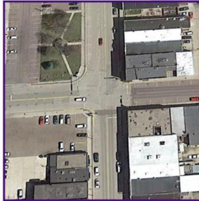
Highway 24 in St. James before construction
