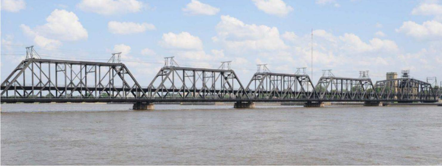
The Government Bridge is a twin-deck structure that accommodates the IAIS rail traffic on the upper deck and vehicle and pedestrian traffic on the lower deck. The roadway portion on the bridge consists of a two-lane public roadway with sidewalks on either side. A vertical clearance of 11'-8" and horizontal geometry at the Iowa approach to the bridge restrict the type of trucks that the bridge can accommodate.
